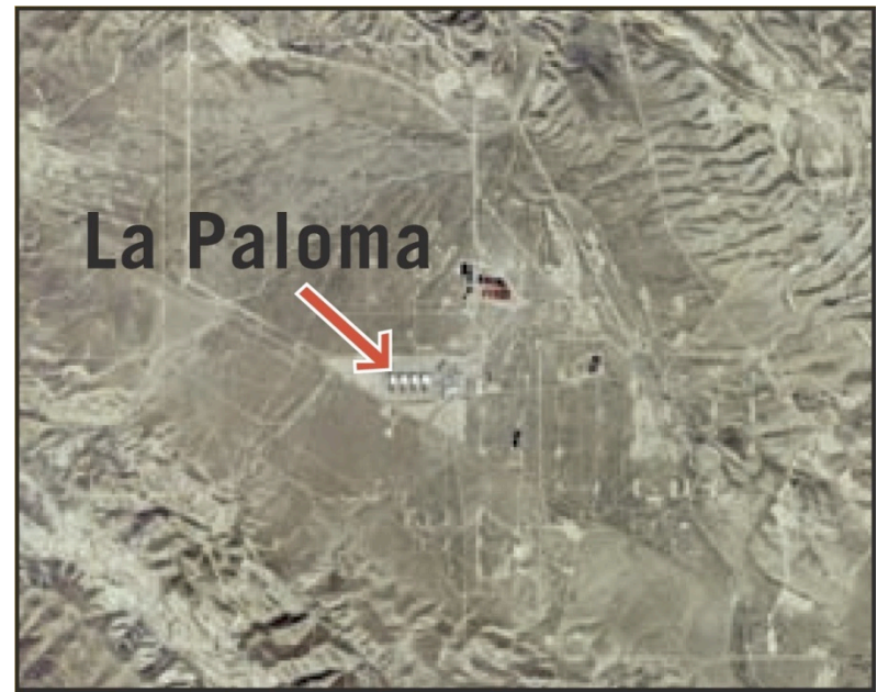
Power plant in a sparsely populated area of California
