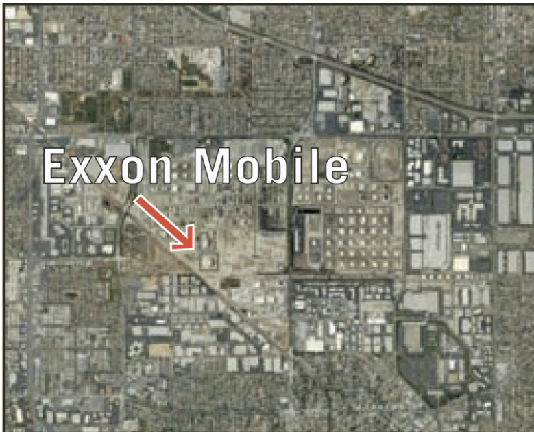
Oil refinery in a densely populated area in Southern California
